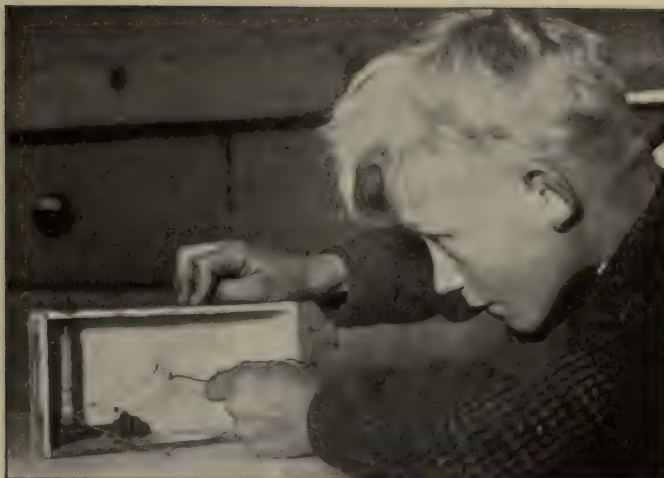
FIG. 139. Sending a message with a cigar-box telegraph.
